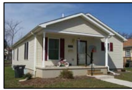
House # 34 September 2007 1131 Charles Street Williamsport PA
