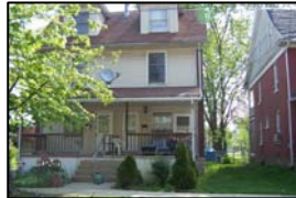
House # 5 March 1993 664 Spruce Street Williamsport PA
