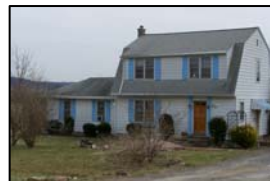
House # 8 September 1996 1312 Ellis Artley Road Pennsdale PA (Rehab Project)
