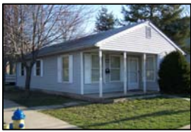
House # 1 November 1990 714 Park Avenue Williamsport PA
